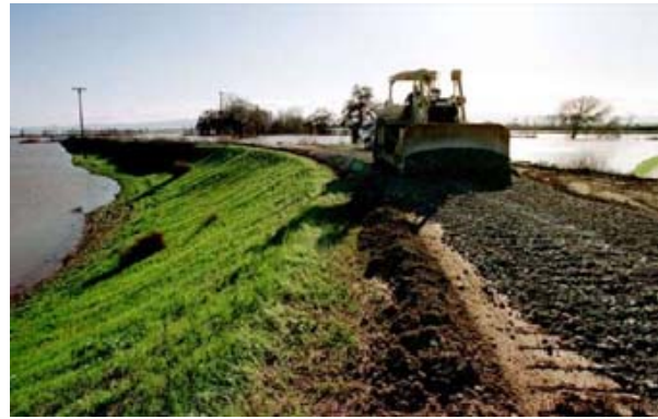
Crown and access road maintenance is performed on a levee.
