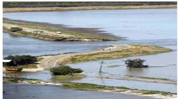
Breached levee
