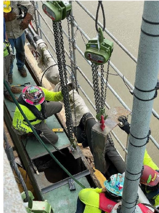
Figure 14. Removal of fractured pieces from tie.
