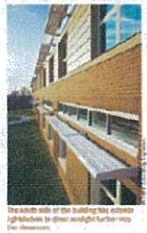
The south side of the building has extra glazing to allow more light for use in classrooms.
