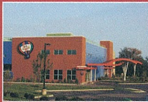
Kaiser Children's Medical Center Hospital with geothermal system Copyright © ASHRAE. All rights reserved.
