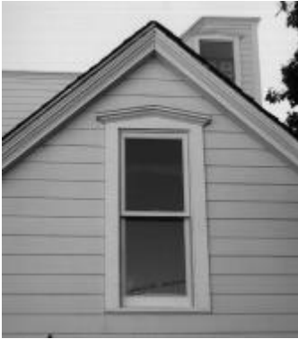
Match a replacement window to the original in its design.
