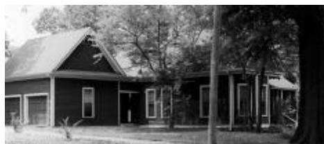
An addition should be compatible in form, scale and materials with the historic building. Using a "connector" to link the new construction with the original is one means of maintaining the character of the primary structure.
