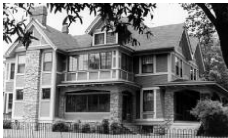
Decorative clapboard siding, multi-paned windows, chimney trim and a hooped metal fence are among the design details that contribute to the character of this property.
