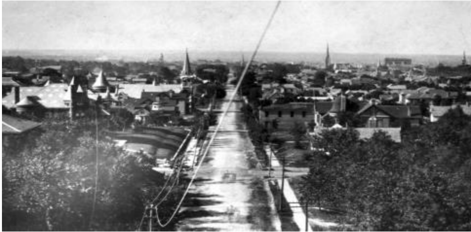
This is a 1890s view looking north from the tower of the Blind School. Churches and grand homes dominated the scene in the early years of what is now the Mansion Area and surrounding environs.
