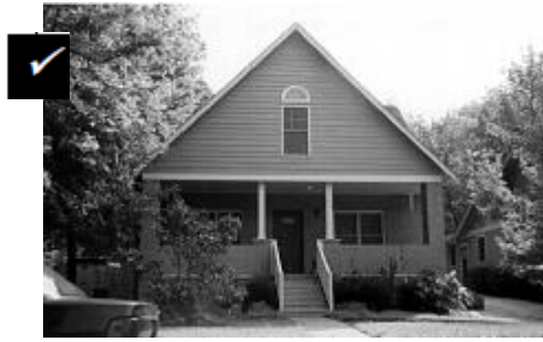
This new infill building appears similar in mass and scale to single-family residences seen traditionally.
