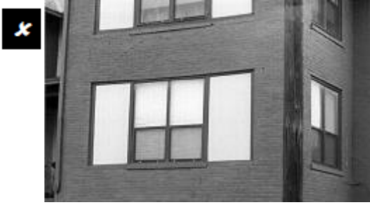
Enclosing a historic window opening on a key character-defining facade destroys much of the building's historic character and is inappropriate.
