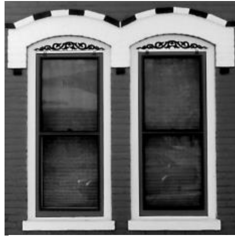
If a storm window is to be installed on the exterior, match the sash design of the original window (as this one does).
