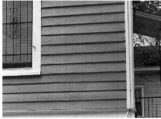
Wood is a typical Little Rock siding and is an appropriate material.
