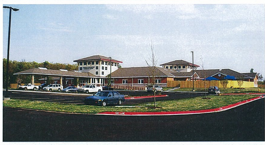
Donald W. Reynolds Emergency Shelter – 42,000 square feet
