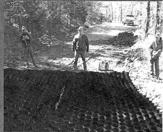
Alternative maintenance practices for stream crossing known as geo-cells
