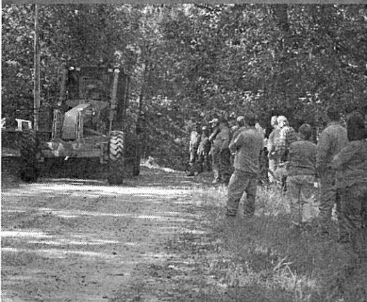
Best Management Practices workshop - Stone county grading demonstration site
