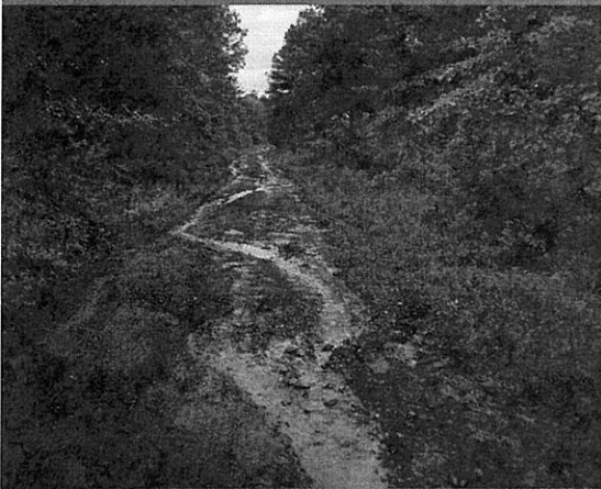
Weak road base material and construction lead to erosion and poor driving conditions
