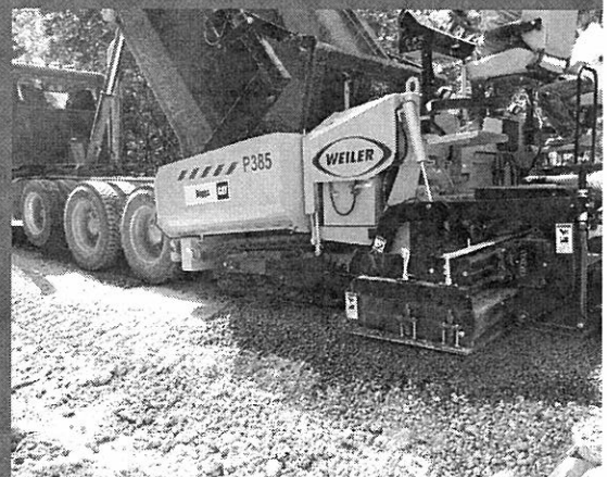
Placing gravel aggregate with a paver
