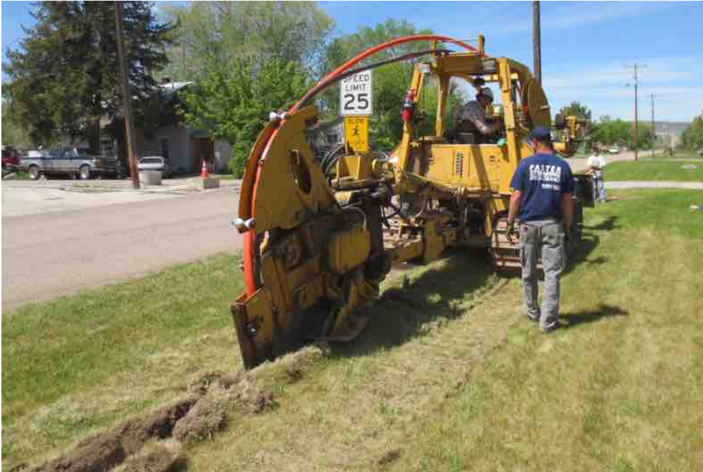
Figure 76. Trenching to Bury Fiber Optic Cable
