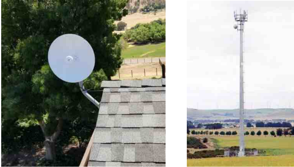
Figure 107. Fixed Wireless Rooftop Antenna and Base Station Tower
