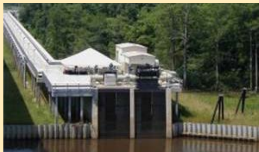
Ouachita River Alternative Water Supply Project intake structure in Union County near El Dorado - Photo courtesy of Union County Water Conservation Board
