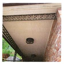
the ceiling was removed, they determined they could do the repairs themselves. The original bead board ceiling was removed and completely replaced.
