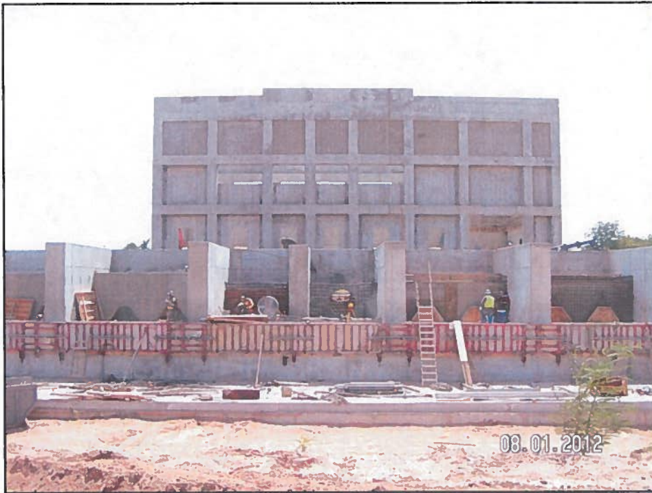
Bayou Meto Pump Station No. 1 splash basin
