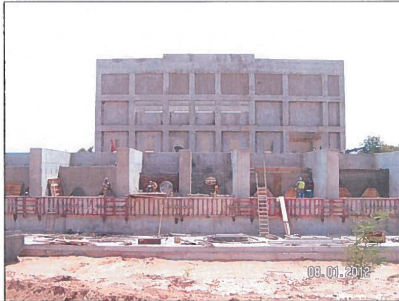
Pump Station No. 1 Construction is 69 percent complete. Completion Date: July 2013
