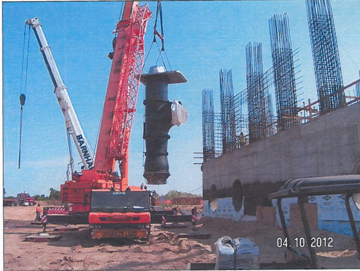
Setting a 186,000 Gallon Per Minute Pump
