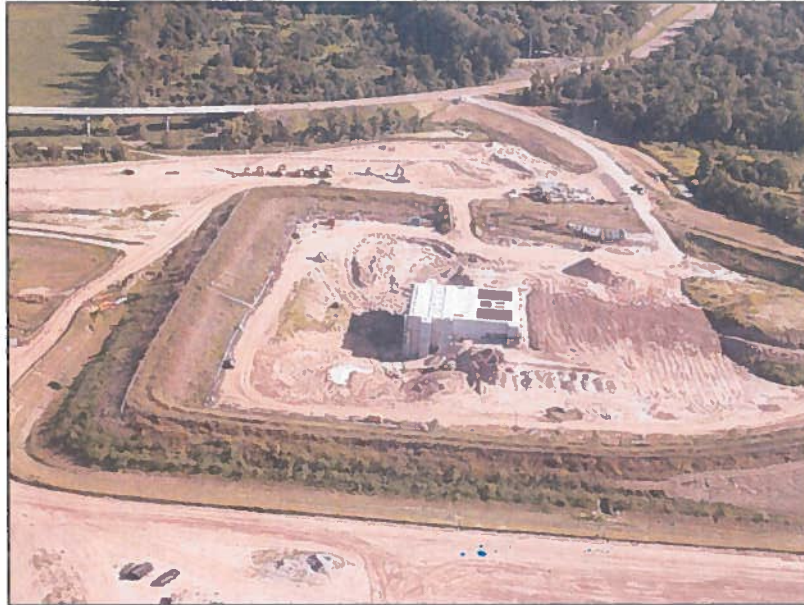
Pump station substructure $9.8 million contract, 79% complete
