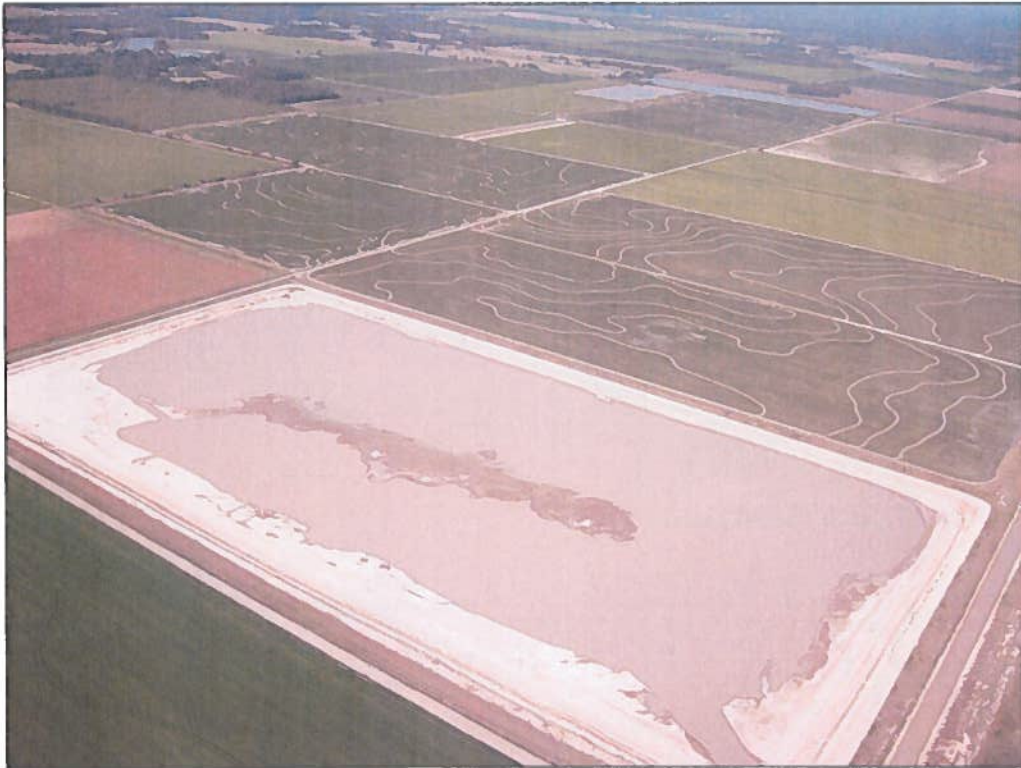
On-Farm storage reservoirs Approximately 250 have been constructed as part of the project
