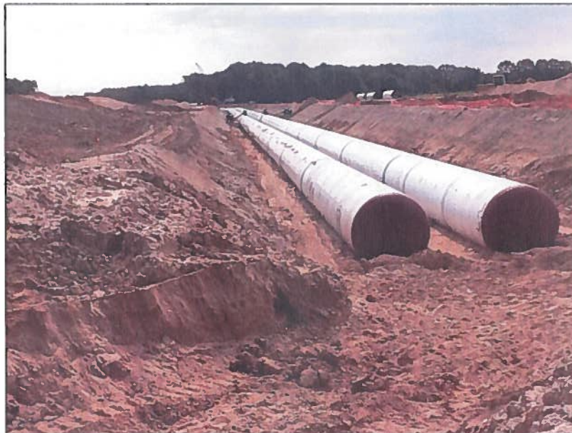
Discharge pipes $10.6 million contract, 98% complete
