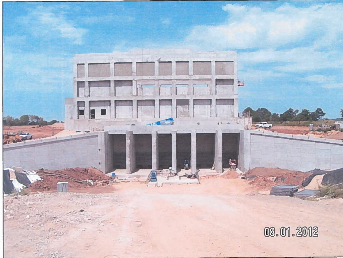
Inlet Channel Bayou Meto Pump Station No. 1
