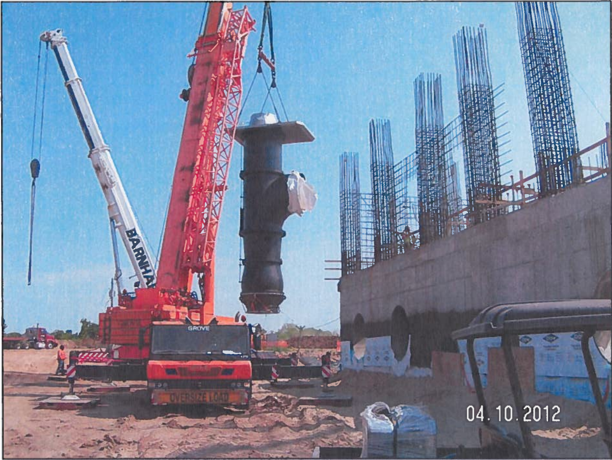
186,000 Gallon per minute pump installation at Bayou Meto Pump Station No. 1
