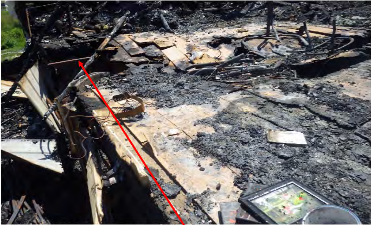
Photo No. 11: View of fire patterns at floor level near front door entrance to residence
