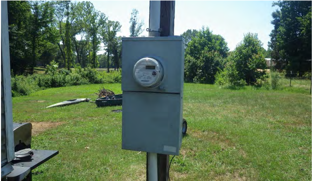
Photo No. 7: View of pole mounted electric meter socket and main breaker for residence
