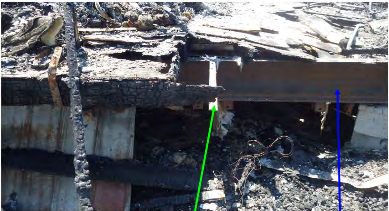
Photo No. 18: View of directional fire patterns at area of fire origin & tempering on steel
