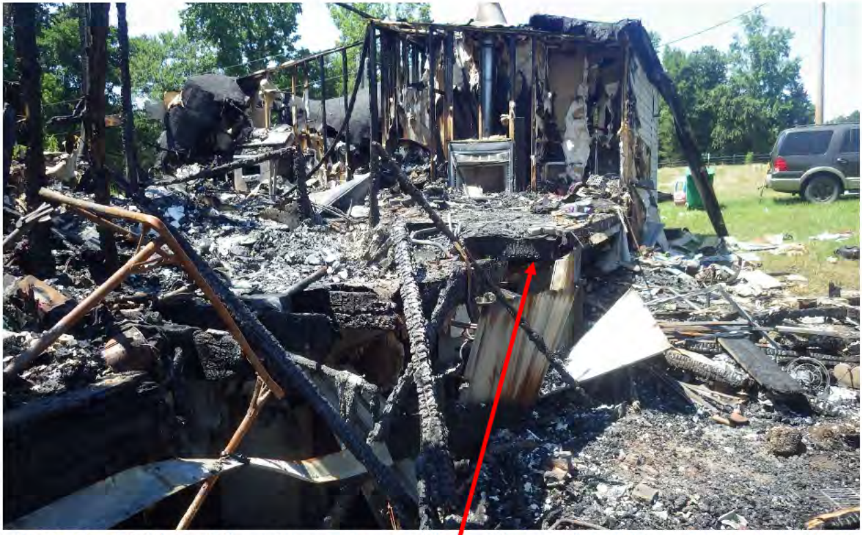
Photo No. 17: View of fire patterns at area of fire origin near front door, note that attached and elevated wood deck is completely burned away
