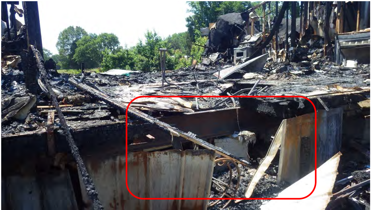
Photo No. 14: View of area of fire origin near exterior side of front door entrance
