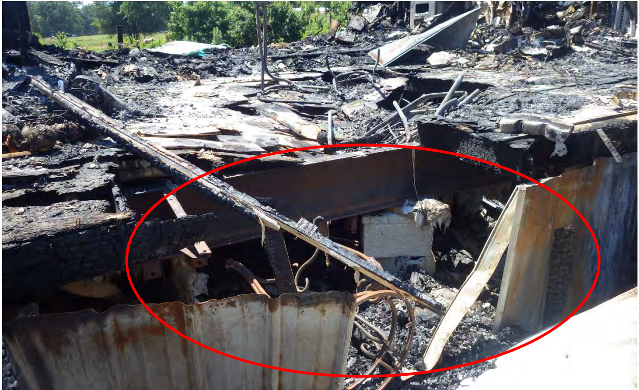
Photo No. 13: View of fire patterns at front door entrance where wood deck was attached to residence, note loss of mass and depth of char on wood framing
