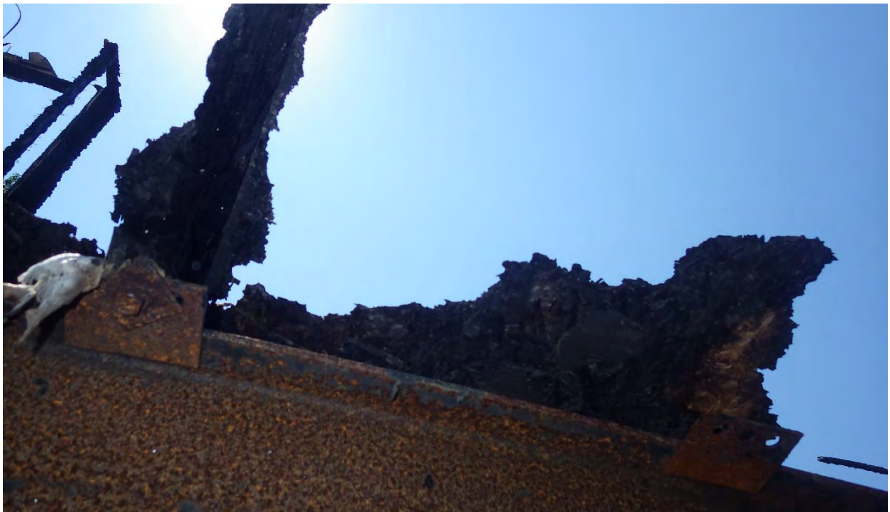
Photo No. 20: View of fire patterns on underside of sub-flooring near front door entrance
