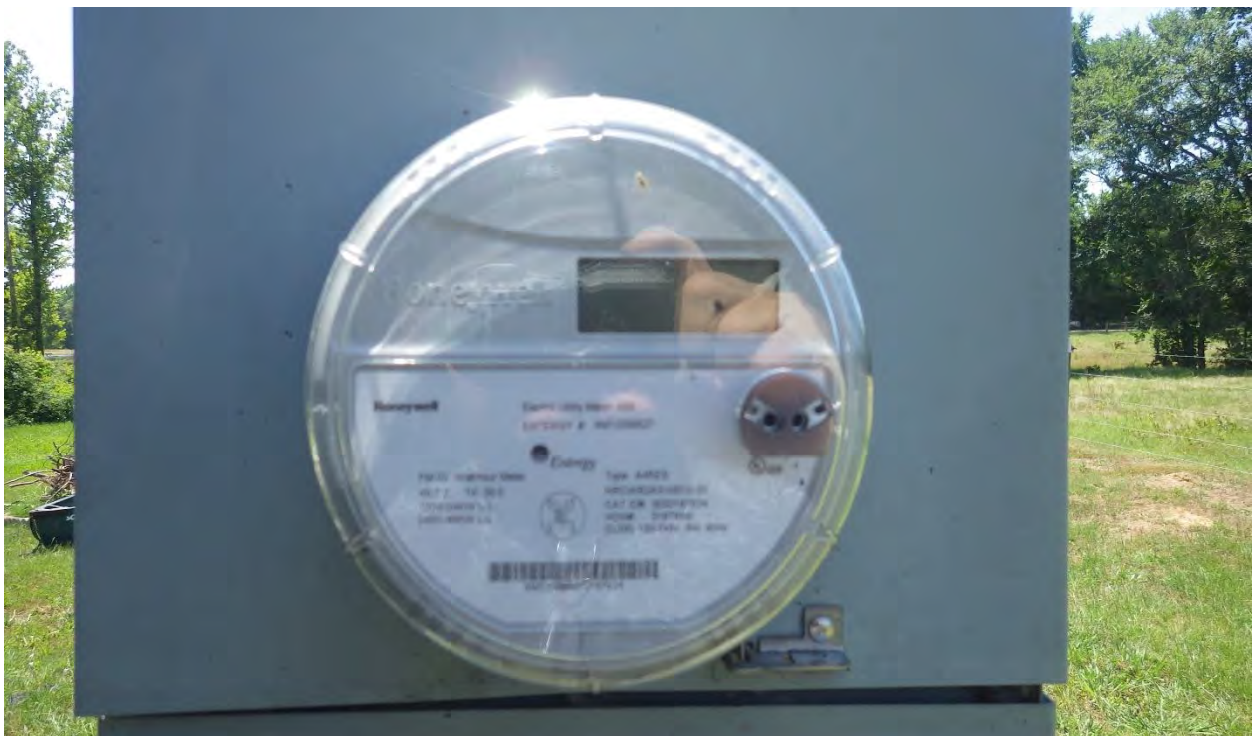
Photo No. 8: View of intact Entergy MDM (smart) meter manufactured by Honeywell
