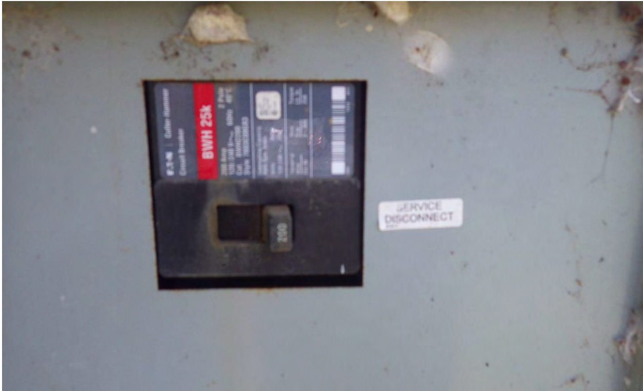
Photo No. 9: View of 200 amp Cutler-Hammer service disconnect breaker
