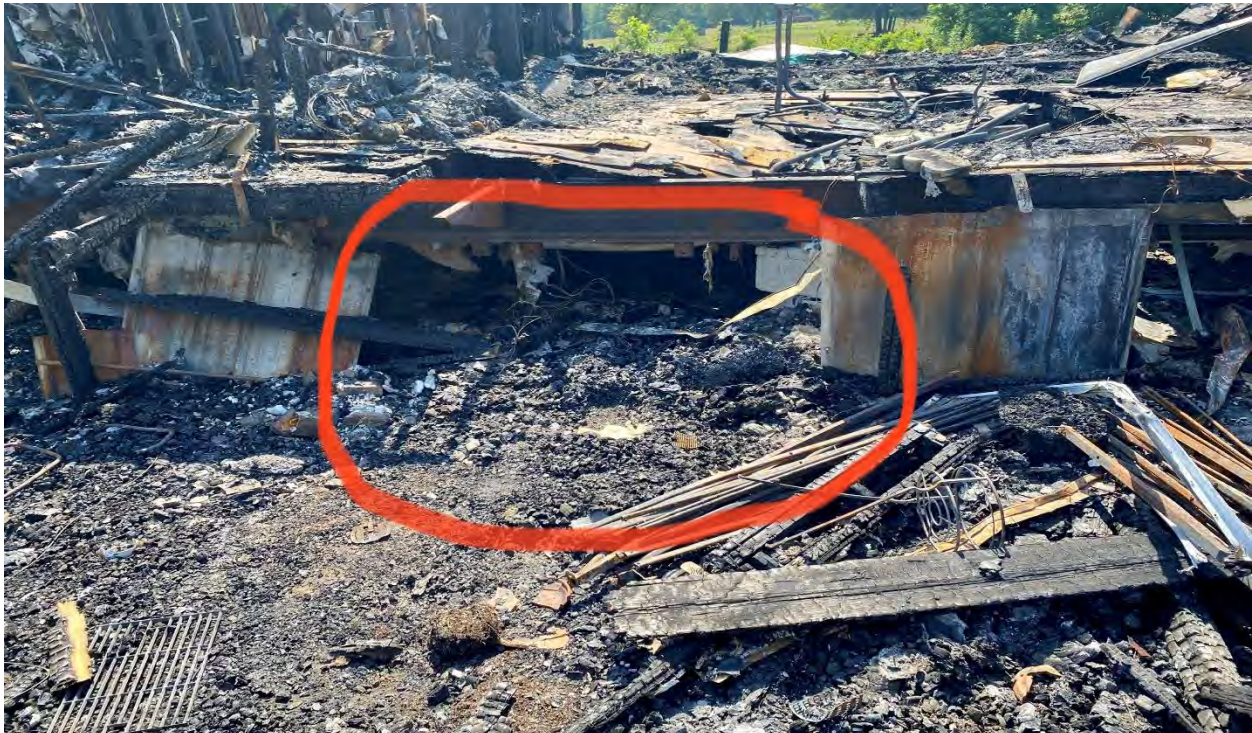
Photo No. 22: View of general area of fire origin on attached wood deck
