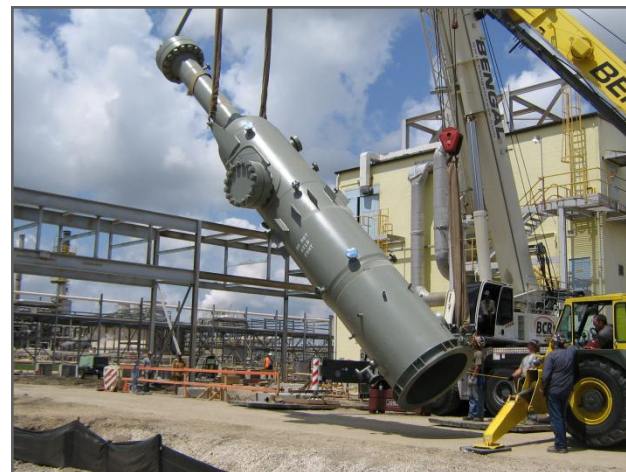
Cold separator installation
