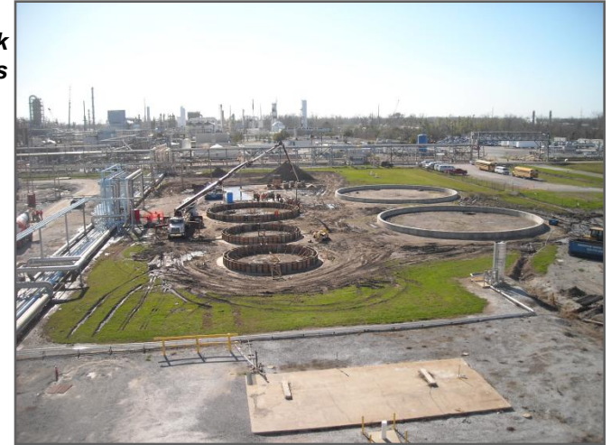
Pouring tank foundations
